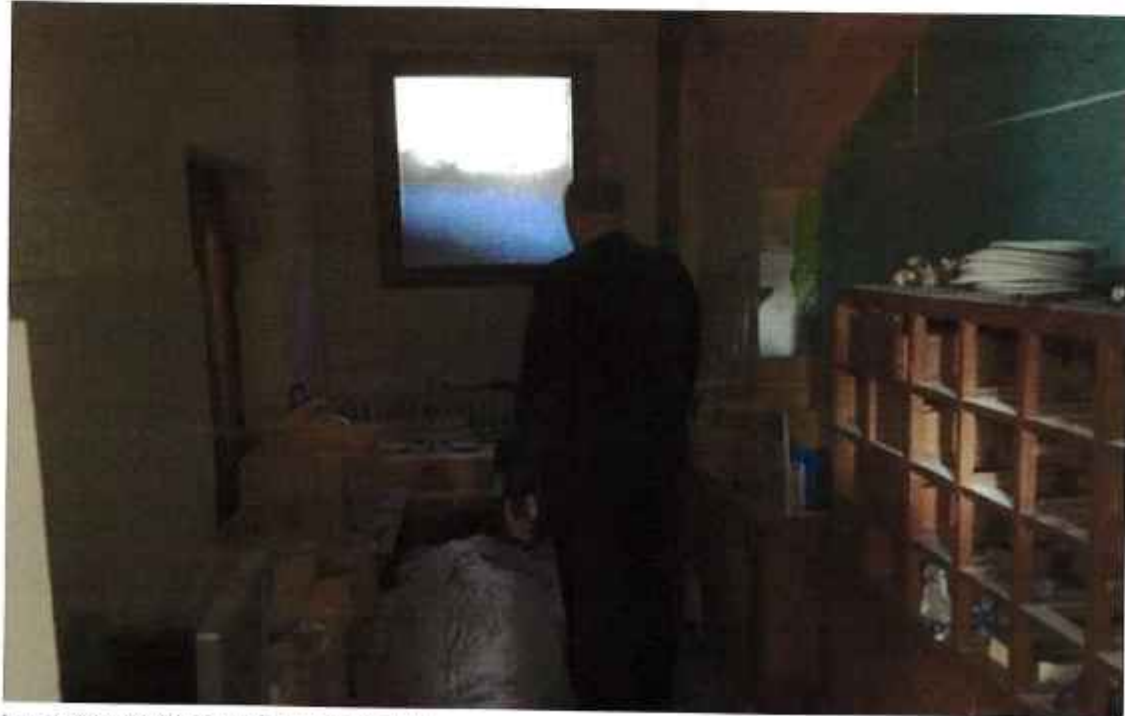
Image no. 18: Sremski Karlovci Grammar School - current condition 1
