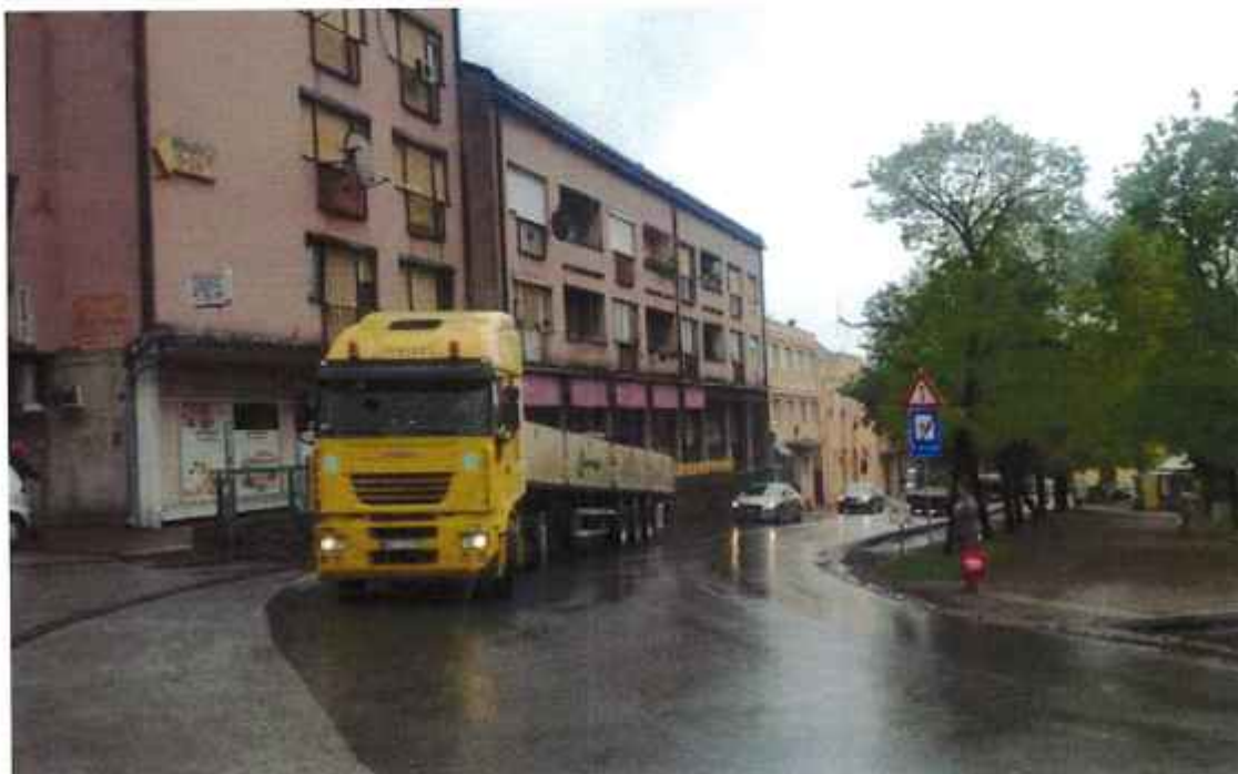
Image no. 30. State road of Ib order no. 21 that crosses the park and central square in Irig - current condition
