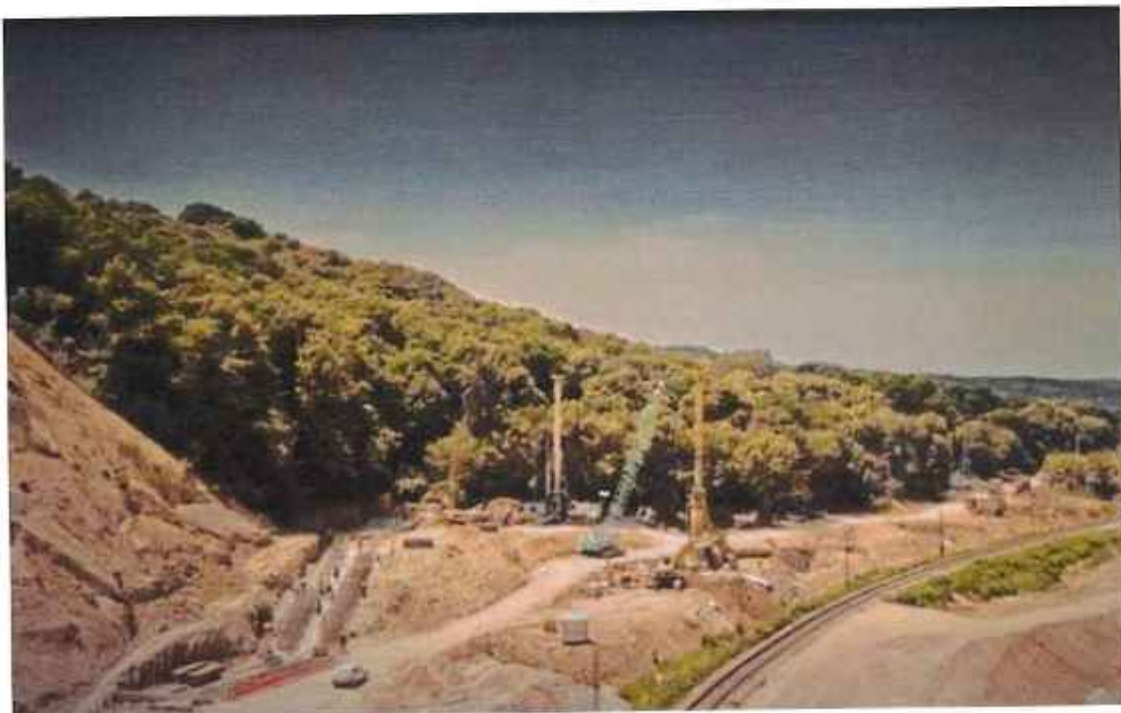
Image no. 1. Construction of railway line - detail no. 1 (Gutanovci)
