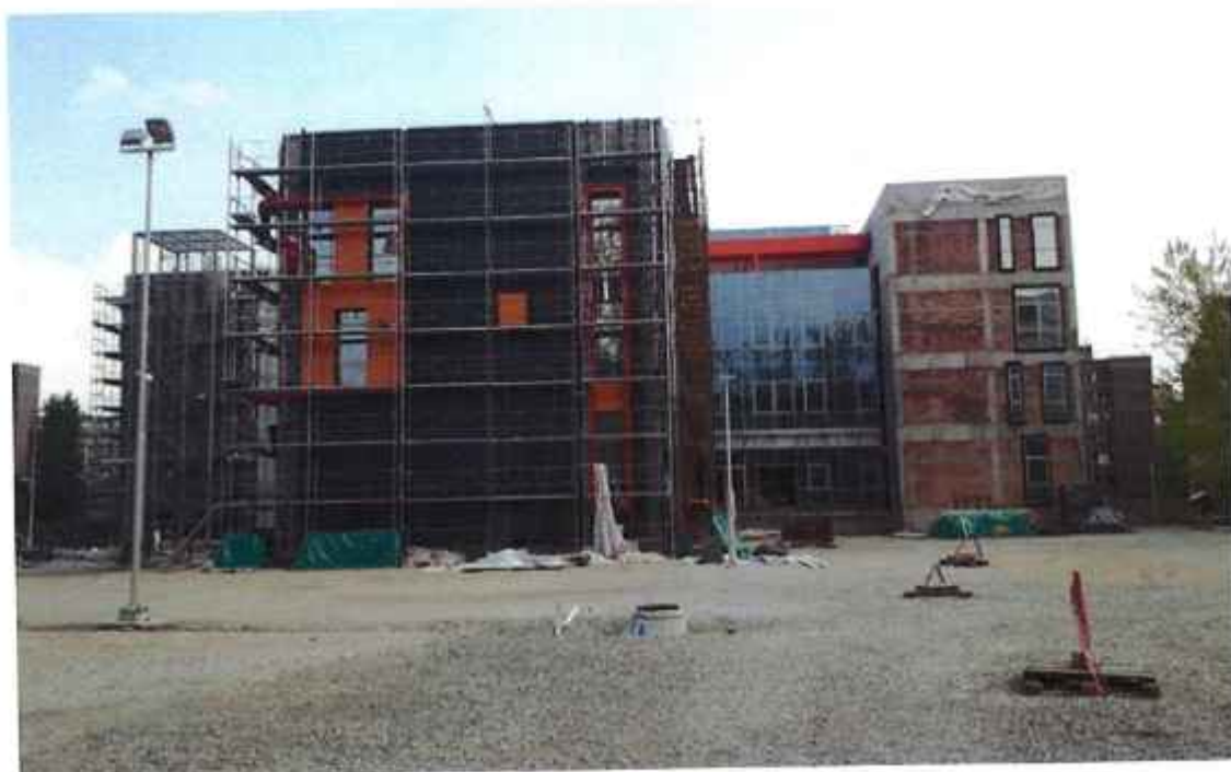
Picture no. 2 Works on the third construction phase.
