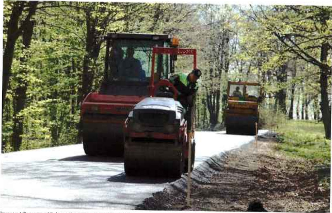
Image no. 4: Restoration of Goleben road – a detail, after the reconstruction
